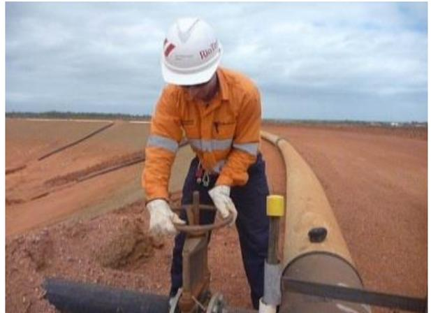
**Figure 1 Manual method previously used to open and close valves**
